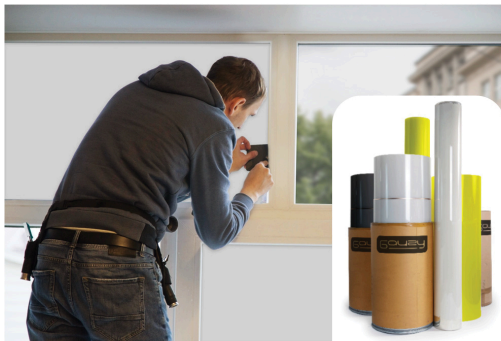
PDLC Retrofit Film Installation; PDLC Film Rolls
